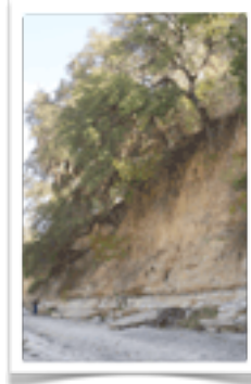
Slowly eroding embankment along the Blanco river
